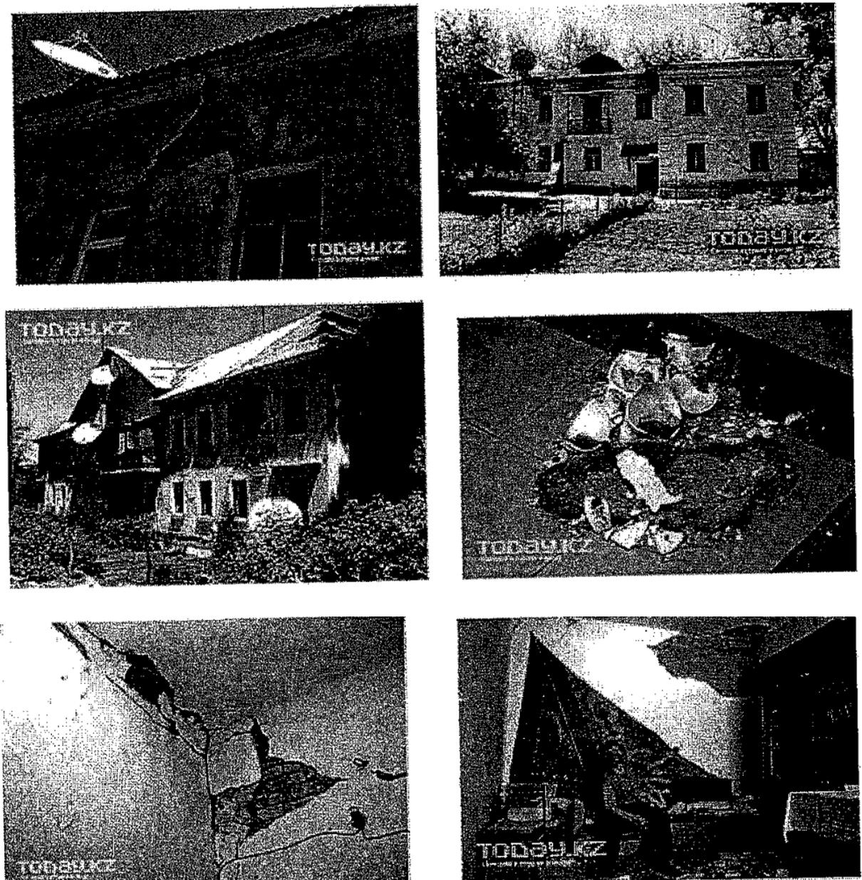
**Figure 1.** Buildings damages in Tekeli town after the earthquake of 13.06.2009 (from [www.today.kz](http://www.today.kz) site)
